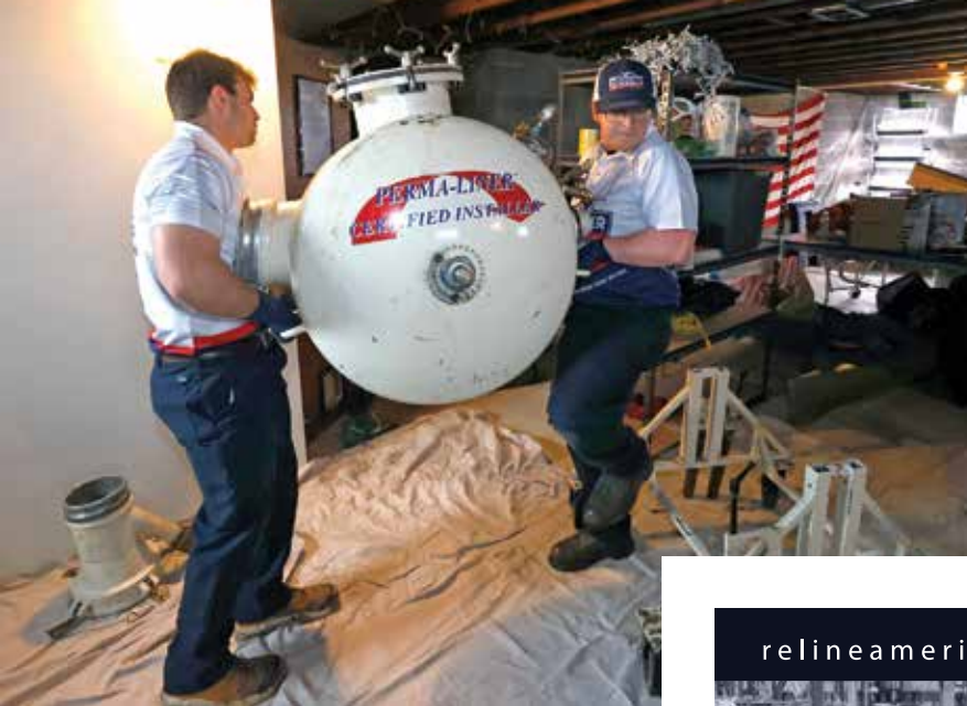
« Gilbert and Murphy move equipment into place for a lining job. Among Hoover's lining tools is a steam-cured system from Perma-Liner Industries.
